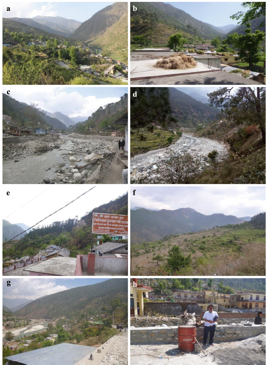
Fig. 24.3 a Bhatwari after Landslide of 2013, b Jamak after Earthquake of 1991, c Gangori after Asiganga (2012) and, d Rawada after Asiganga Flash Bhagirathi (2013) Flash flood, e Pata after Varunavat, f Sangrali after Varunavat Landslide (2013), g Mandon after Forest fire, h Reconstruction by community Asiganga and Bhagirathi Flash flood members of Tiloth after flash flood (2013), i Embankment formed in Joshiyara, j Landslide zone between after Flash flood (2013) Dharasu and Nalupani
